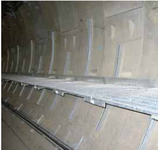
Fastening on curved framing channels
