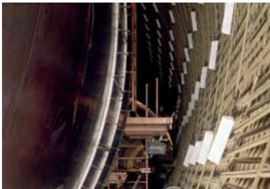
Fastening the anchor channels to the formwork
