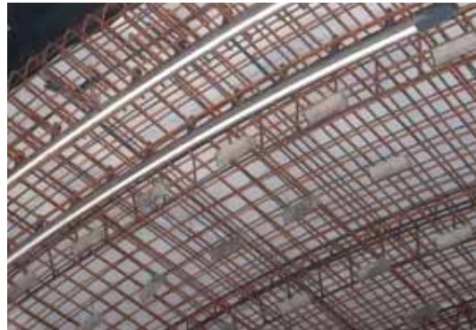
Fastening the anchor channels to the reinforcement
